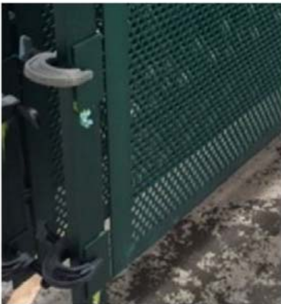
CLAMP MARK ON CUTOFF TAB REMOVED BY CLIENT AFTER ANODISING AND TOUCHED UP.
